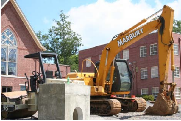
Installation of drainage system
